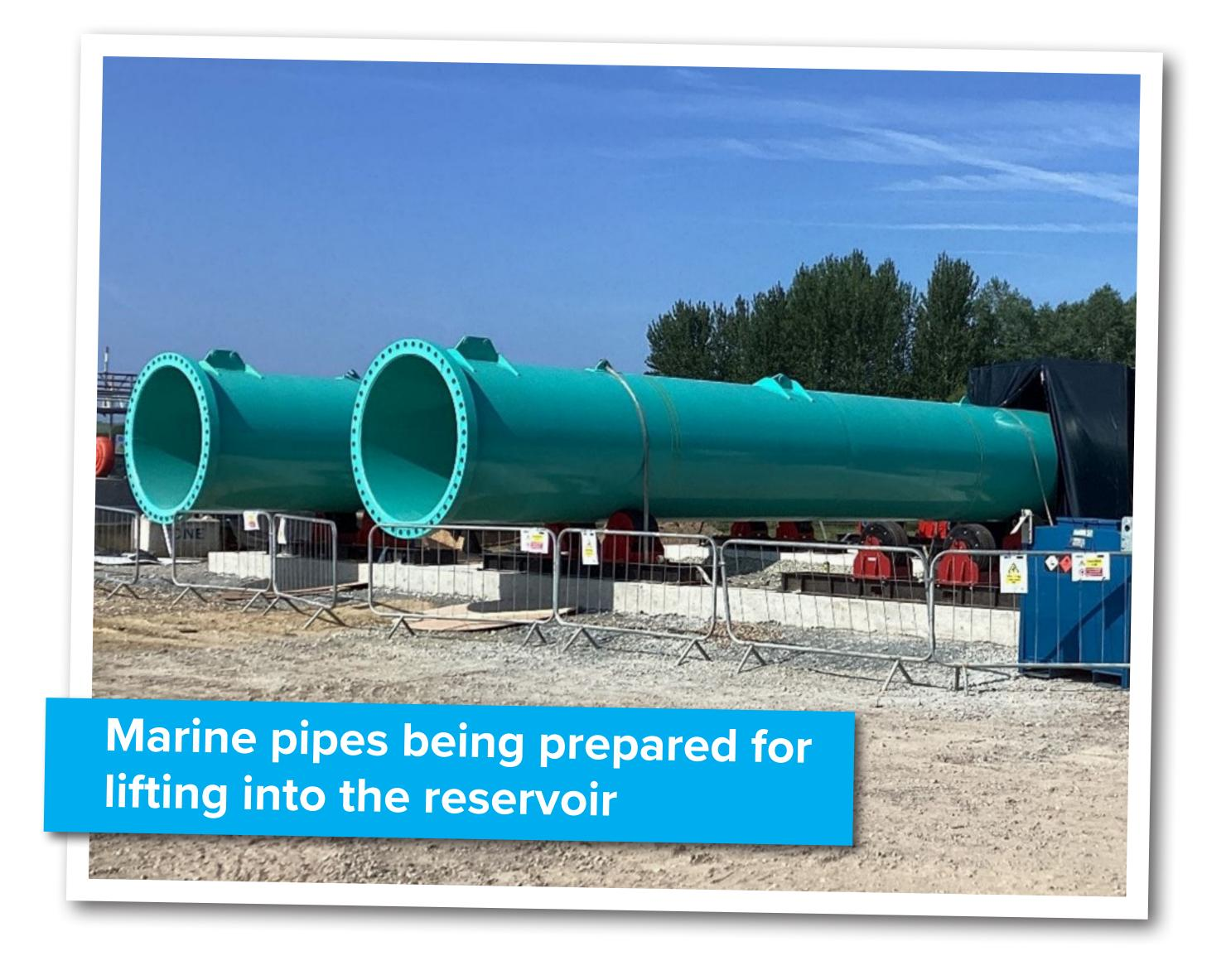
The pipes will be stored in the reservoir until October while we prepare the dam's protective surface. Once this is complete, the pipes will be floated into position on the upstream side of the dam and lowered into underwater supports in a complex operation involving floating pontoons, trolley systems, winches, and specialist divers.
