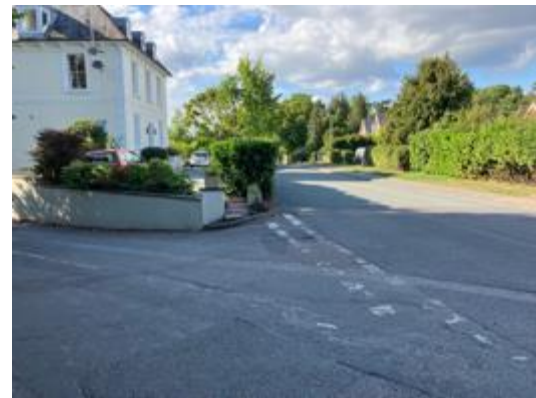
Picture 2 – Tapsells Lane junction onto Station Road is a dangerous junction
