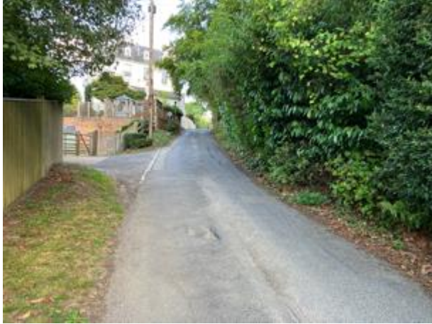
Picture 3 – Tapsells Lane towards Station Road - dangerous for pedestrians as it has no street lighting or footways
